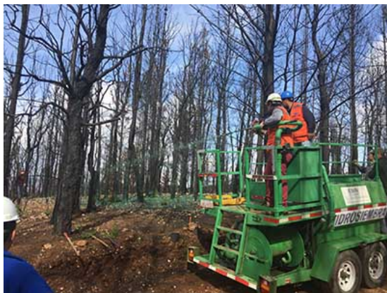
Hydro-seeding, International Erosion Control Association
